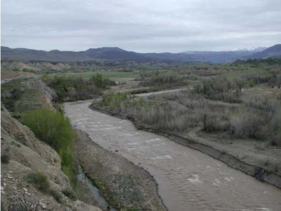
USACE Site 3: Channel alteration, reduced sinuosity, reduced vegetative cover, bank instability
