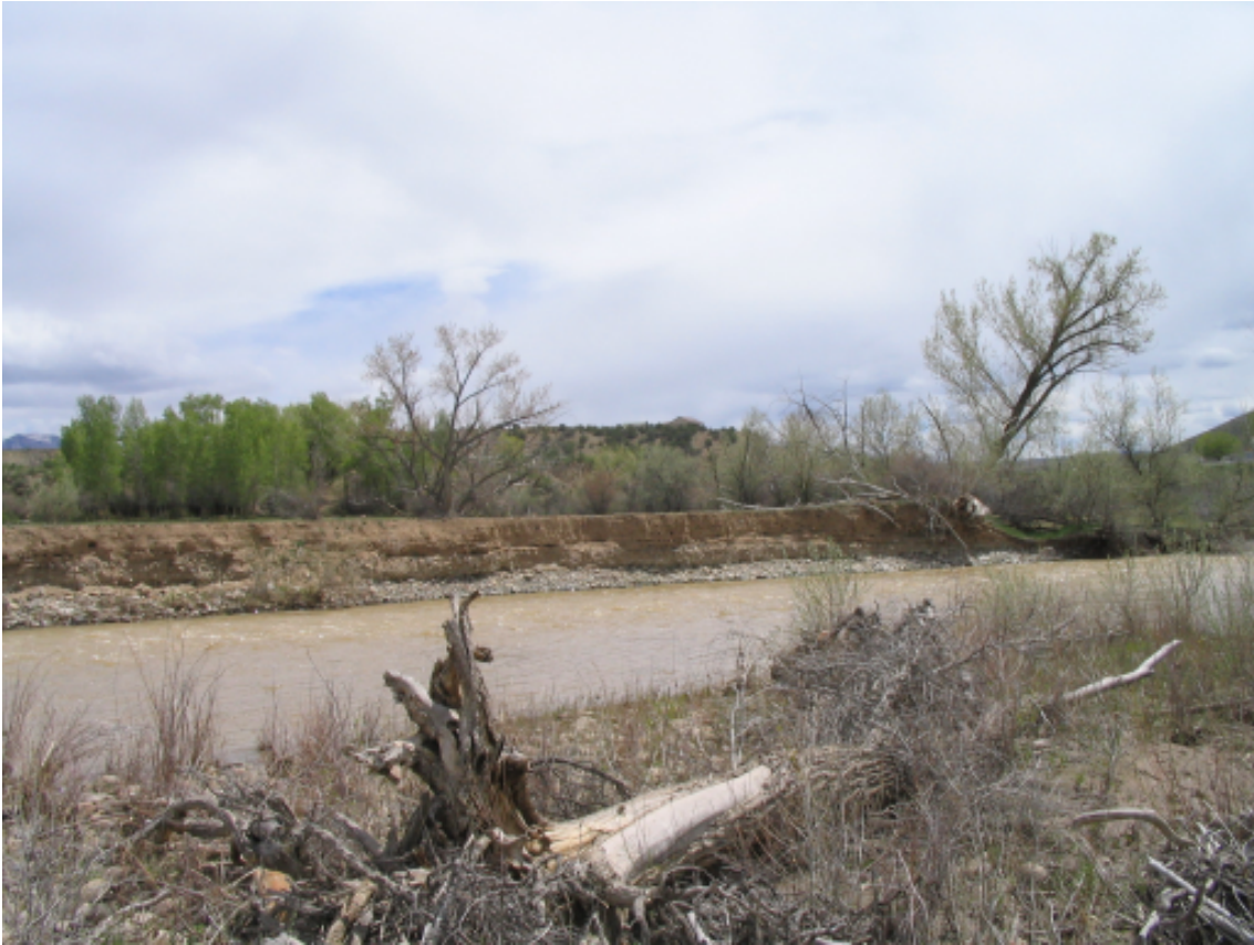
USACE Site 2: Bank erosion and sloughing adjacent to bank (channel widening, loss of bank vegetation)
