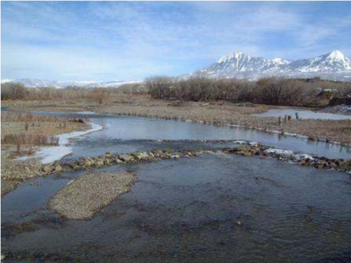
Completed low-head rock weir just above Smith-McKnight Ditch site on Hwy 92 in Hotchkiss
