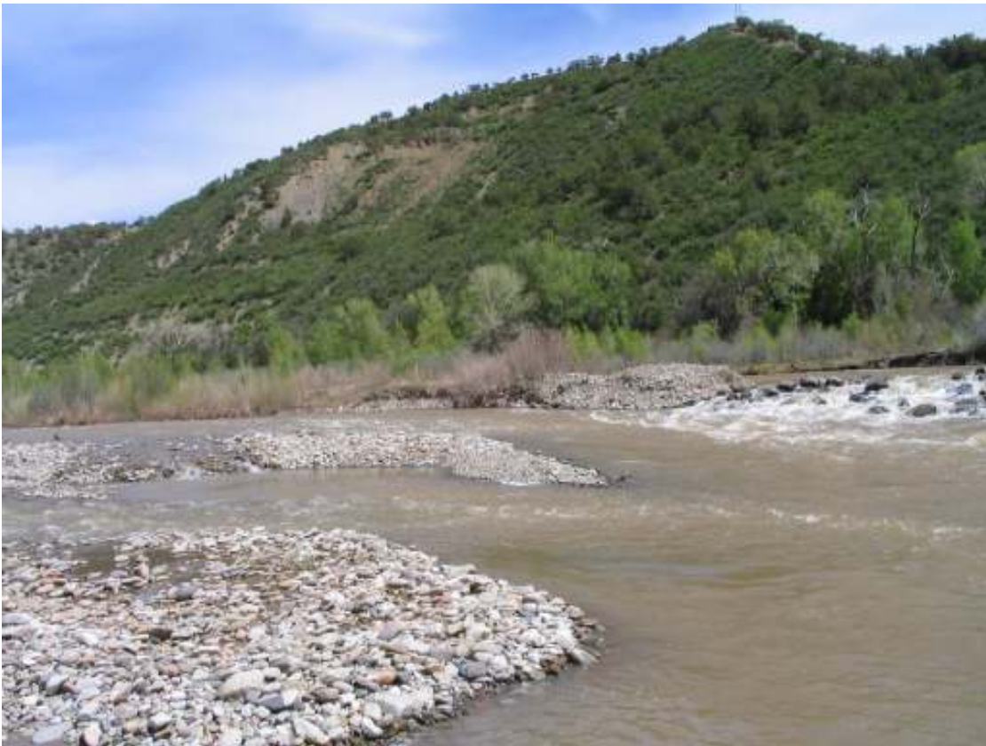
Stewart Diversion: Irrigation diversion dam, localized channel erosion, annual maintenance - bed and bank disruption.
