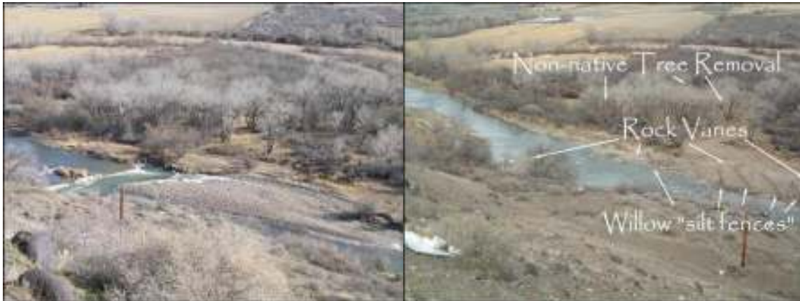
Chipeta dam site before and after restoration
