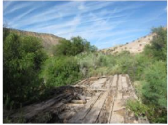
FIGURE 0-21: LOOKING WEST AT OLD WOOD PLANK BRIDGE. BLM GUNNISON GORGE WILDERNESS AREA BEGINS AT THIS POINT (07-10-15)
