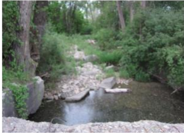
FIGURE 27: OLD DAM AND DIVERSION STRUCTURE ON SMITH FORK BELOW CLIPPER DITCH (07-18-16)
