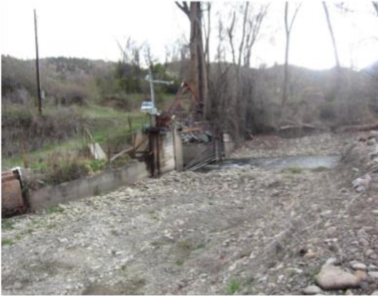
FIGURE 0-17: CLIPPER DIVERSION: DRY BED IN FOREGROUND WHERE GRAVEL WAS PUSHED TO DAM THE SMITH FORK MAIN CHANNEL TO CREATE A BYPASS (04-22-15)
