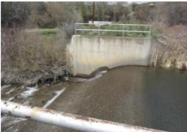
FIGURE 0-13: FEEDER CANAL DIVERSION ON THE MAIN SMITH FORK (04-22-15)
