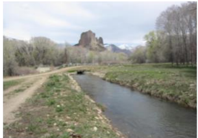
FIGURE 0-14: SMITH FORK FEEDER CANAL CARRIES WATER DIVERTED AT THE FEEDER CANAL DIVERSION TO CRAWFORD RESERVOIR (04-22-15)
