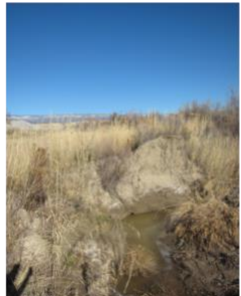
FIGURE 0-10: TONGUE CREEK BANK EROSION AND DOWNCUTTING
