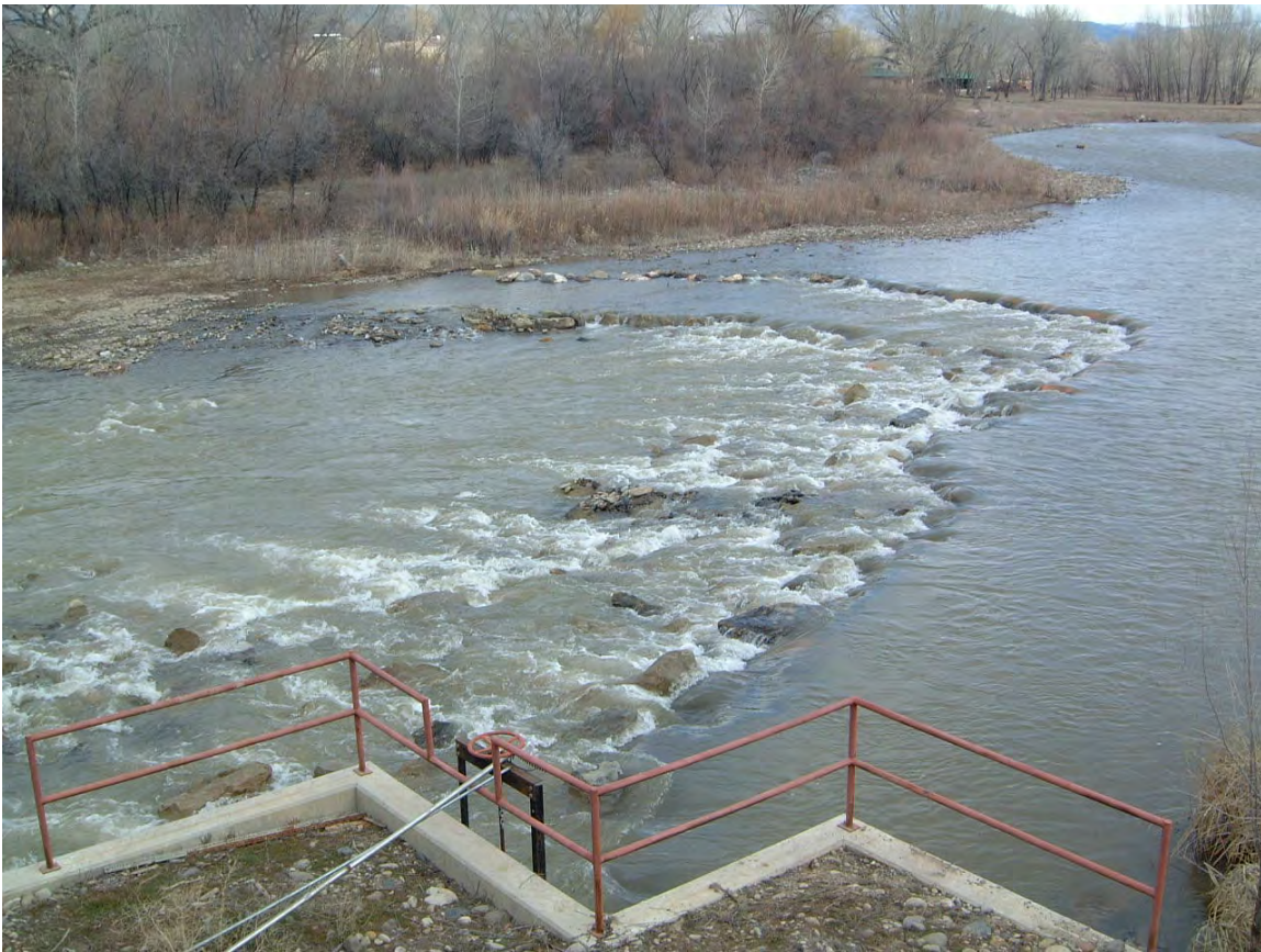
Photo 13. Smith-McKnight Ditch Immediately Following Construction, 2000
