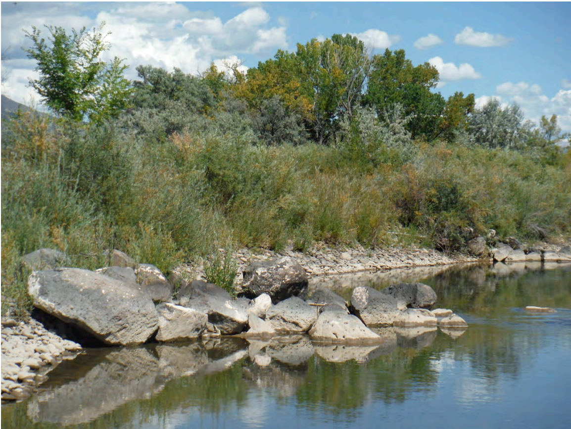
Photo 23. Midway Project: Ross Property Rock Vane, 2014
