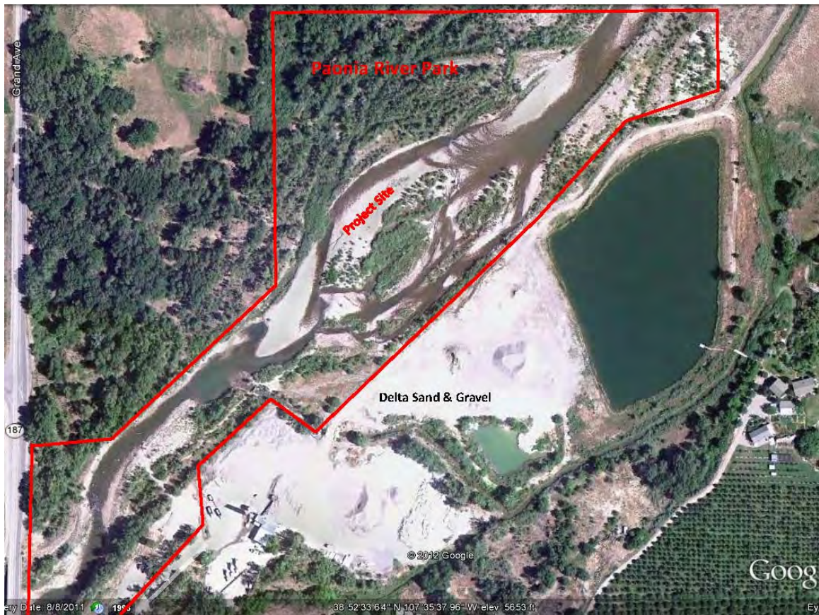
Photo 40. Paonia River Park Site Prior to Construction
