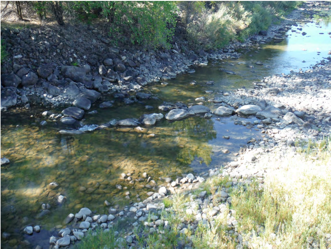
Photo 39. Paonia Sewer Crossing "W" Weir, 2014
