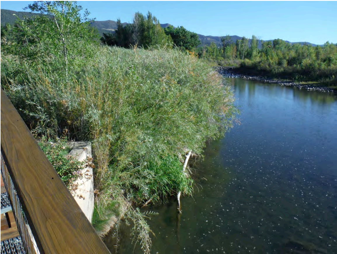
Photo 35. Bank on Monitor Ditch Site, 2014
