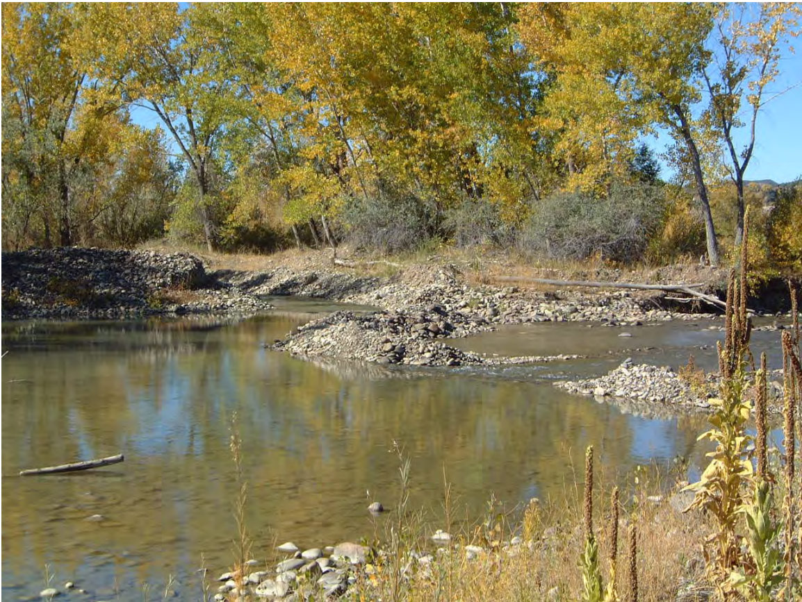
Photo 30. Short Ditch Prior to Construction
