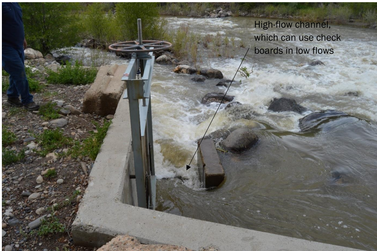
Figure 2.5.2.4. Concrete Headwall with High Flow Channel at Paonia Ditch Intake Structure
