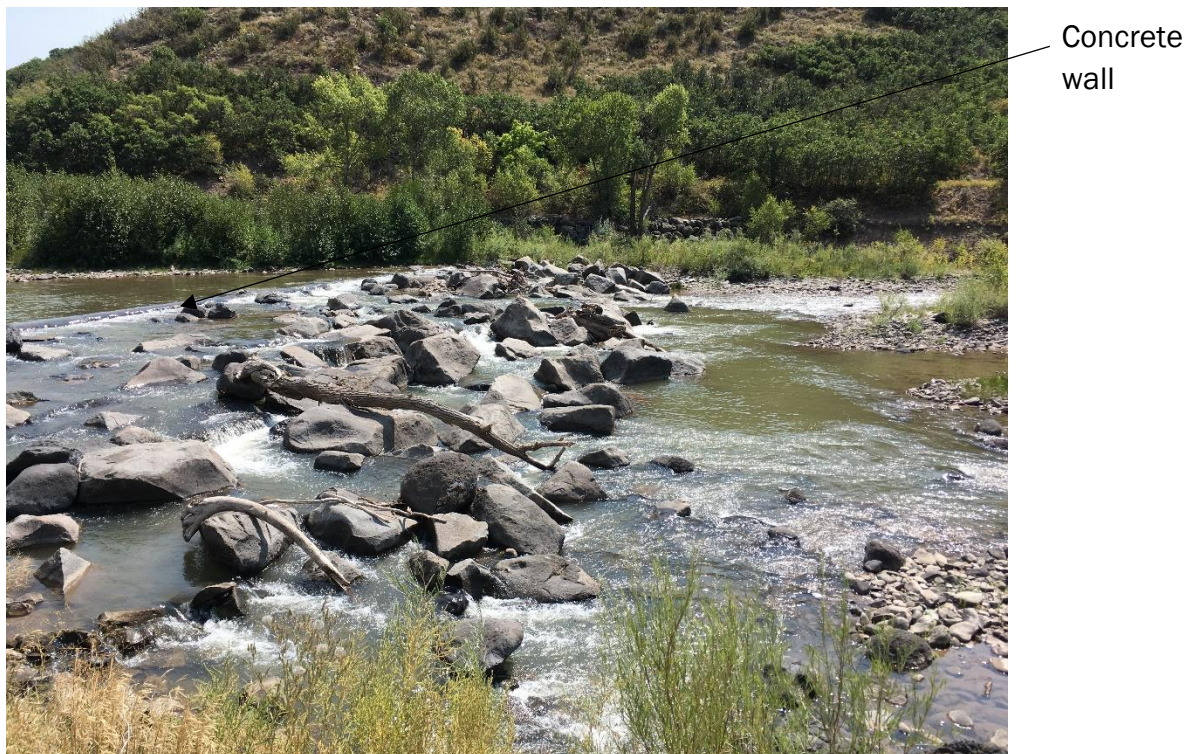
Figure 2.2.1.3. Portion of Concrete Wall with Boulder Backfill
