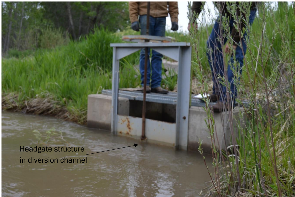
Figure 2.5.2.6. Monitor Ditch Headgate
