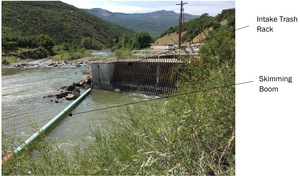
Figure 2.2.1.4. Fire Mountain Canal Intake Structure
