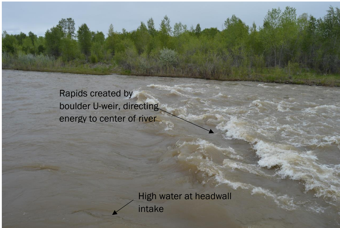
Figure 2.5.2.3. Resultant Water Profile from Monitor Ditch Diversion
