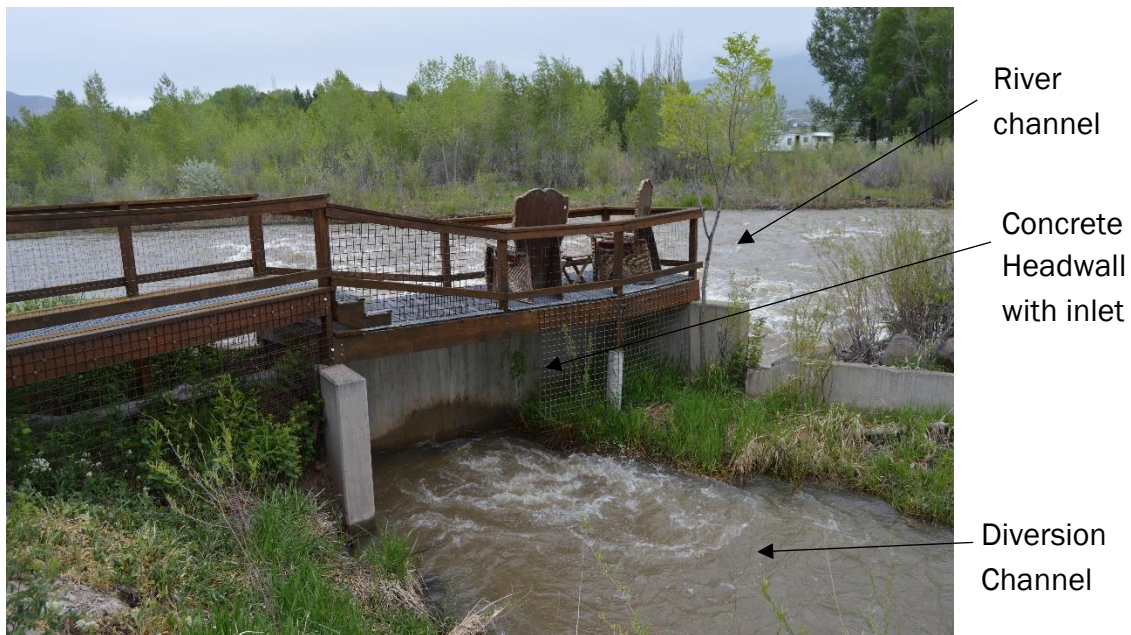
Figure 2.5.2.4. Concrete Headwall for Monitor Ditch at River Diversion
