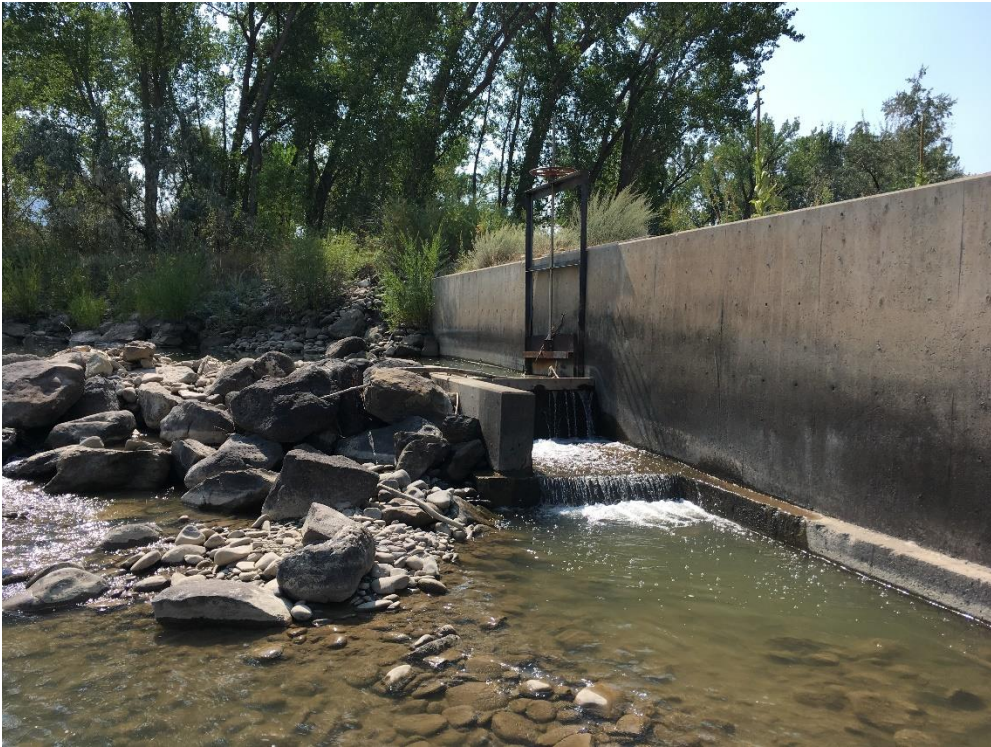
Figure 2.6.1.4. Short Ditch Diversion Headwall and Intake
