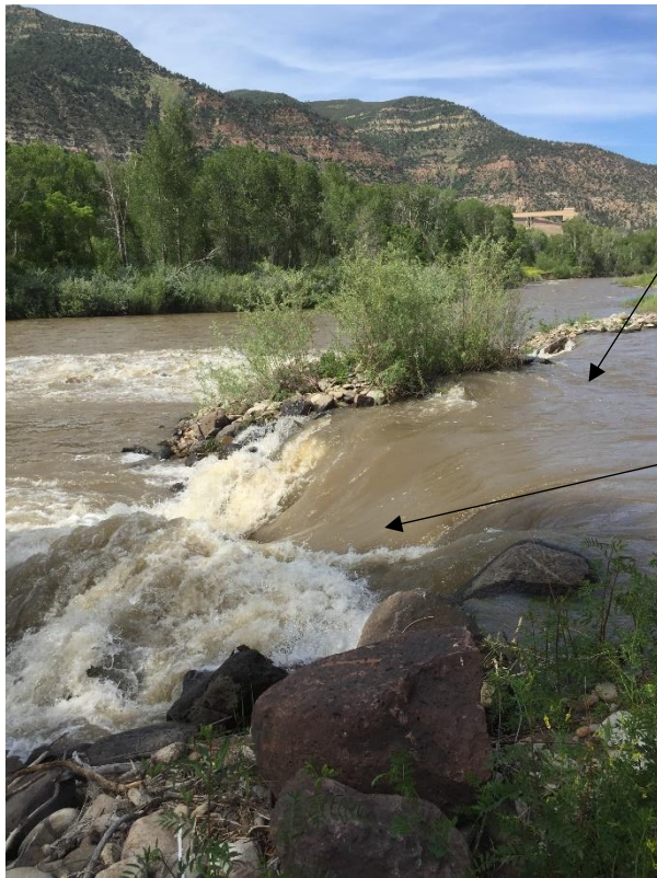
Figure 2.3.1.4. Spill over Boulder Weir
