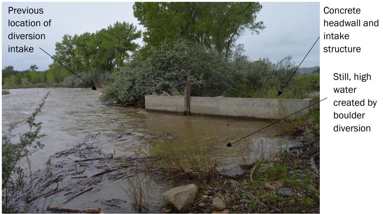
Figure 2.5.3.3. Concrete Headwall and Intake Structure for the Shepherd and Wilmott Diversion
