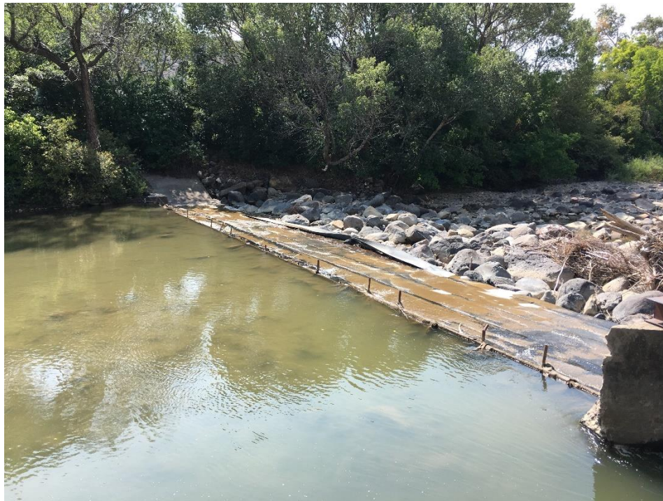
Figure 2.4.1.4. North Fork Farmer's Ditch Diversion
